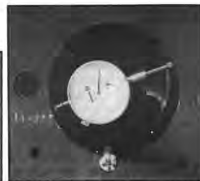
When bellhousing alignment is complete, tighten the set screws to secure the dowel pins for future reassembly without the hassles of realignment.
